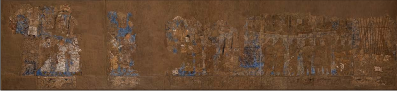
Figure 3. West Wall (Before Restoration)
